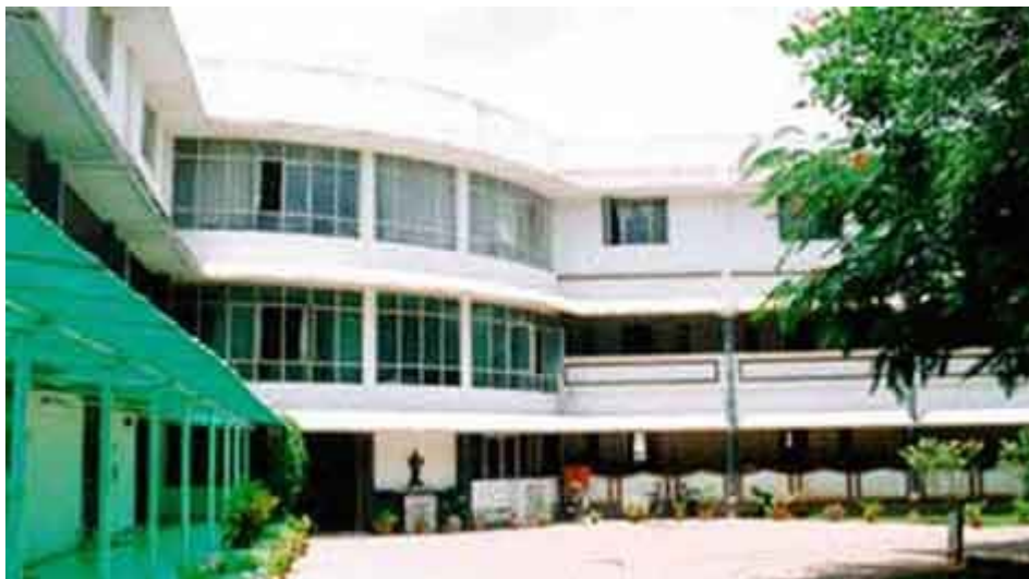
The main reception and part of the clinic complex
